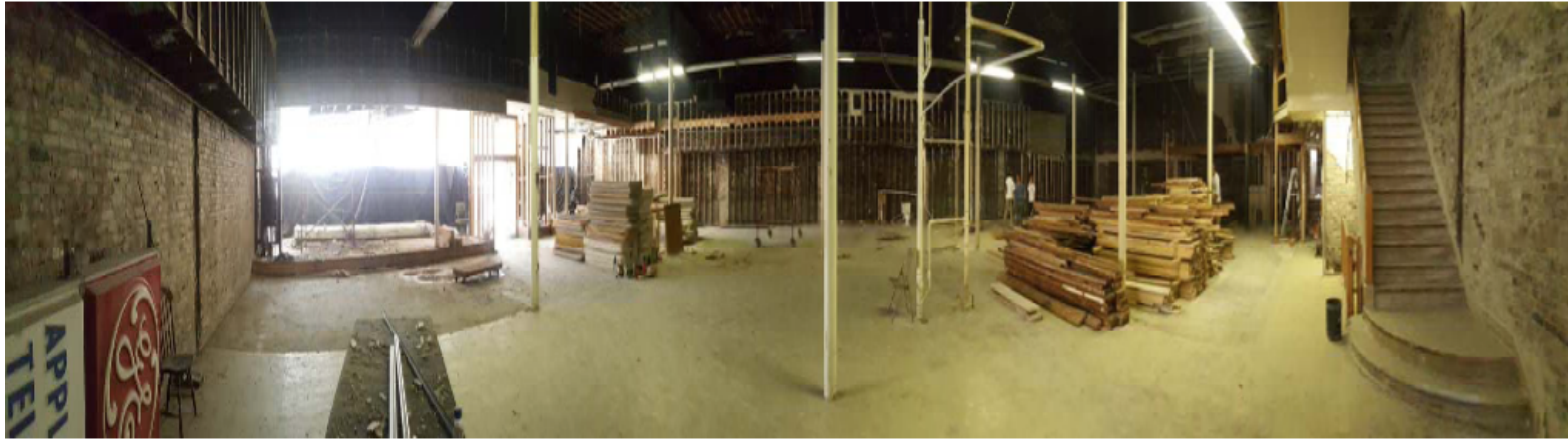
Distorted panoramic view inside the Belk building after demolition started.
